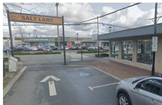
Accessible Parking Space on Salt Lane
