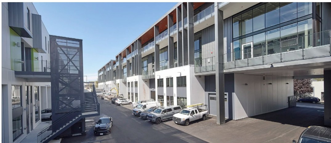
Figure 32 - Locate loading docks and utility areas at the rear of buildings away from pedestrian areas. Source: Ventana. Ironworks (2019). https://www.ventanaconstruction.com/commercial-industrial/ironworks
