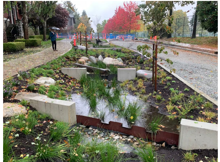
Figure 39 - Bioswales and rainwater gardens are encouraged for stormwater management. Source: Cherie Xiao, City of Vancouver
