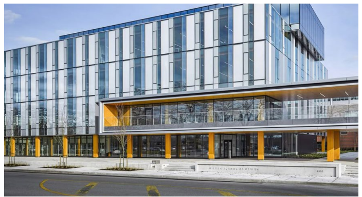
Figure 42 - Create a unique architectural identity with high quality design and materials for the Hub building which includes an active frontage to the 203A Street plaza and park.
